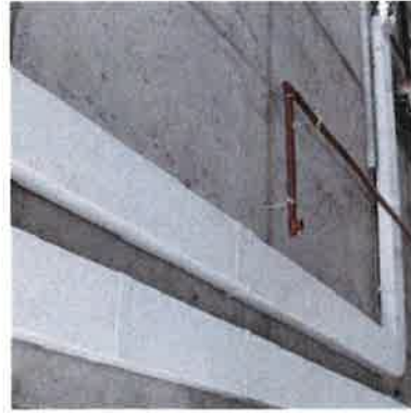
TYPICAL WEATHERPROOF LOUVRE DETAIL C/W FLAT DUCT CONNECTION BEHIND
