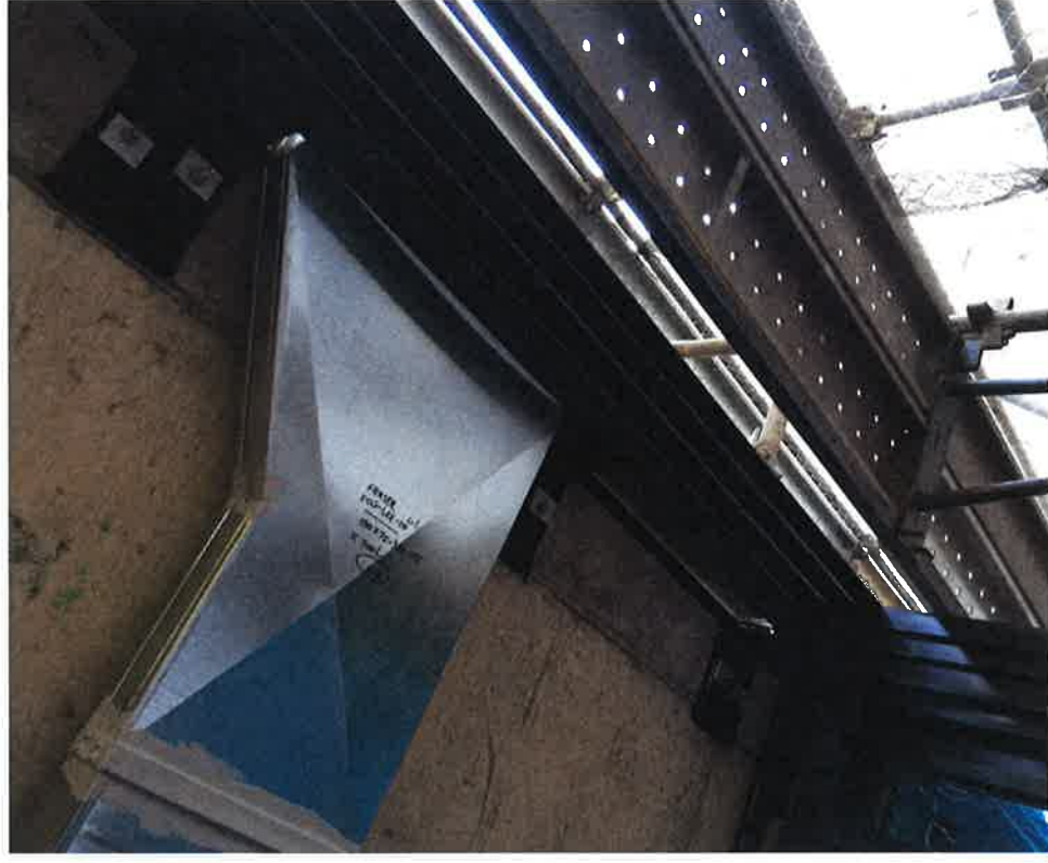
ALTERNATIVE FABRICATED SLIMLINE DUCT
